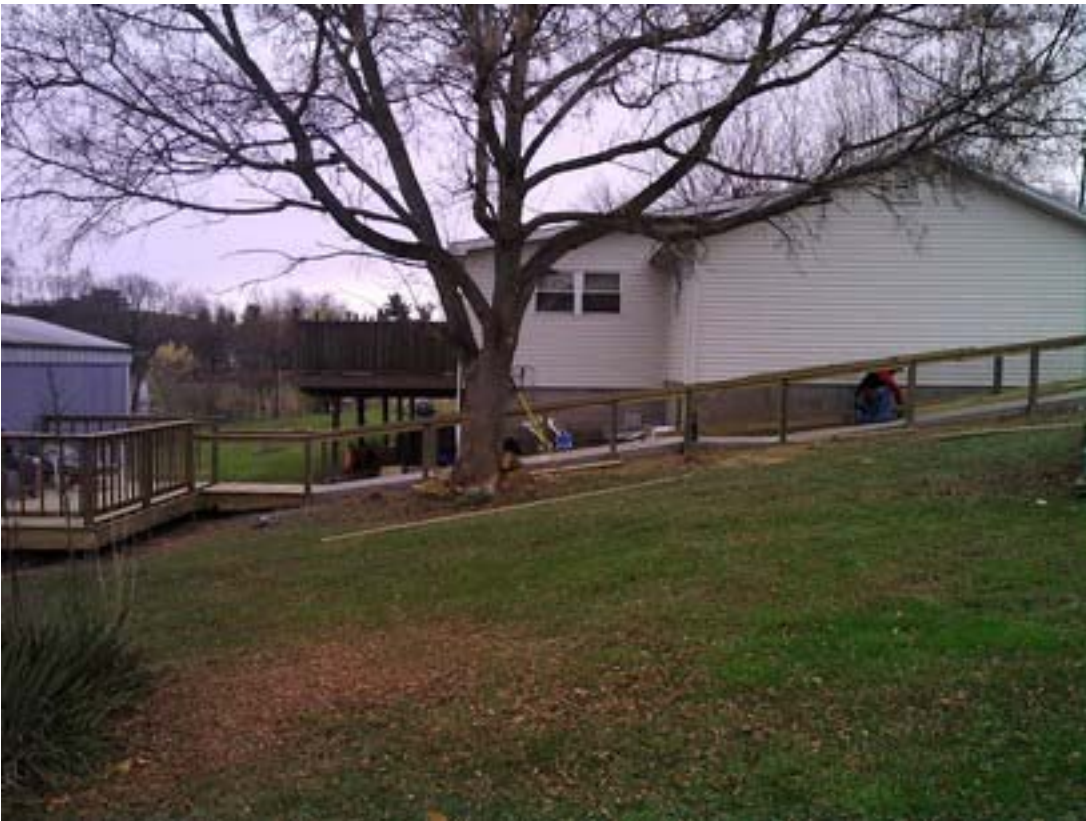
Figure 4 A long concrete ramp. Brushed concrete is required for these applications; notice the landing in the middle of the ramp.
