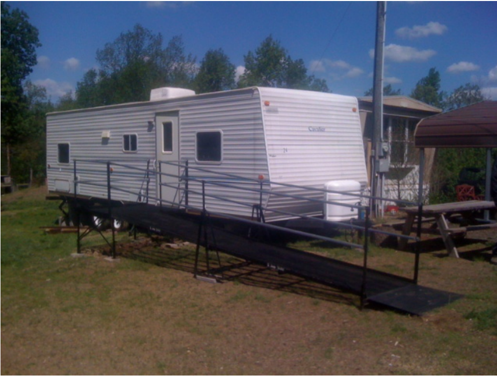
Figure 1 A metal ramp, the bottom rail is integrated into the ramp surface.
